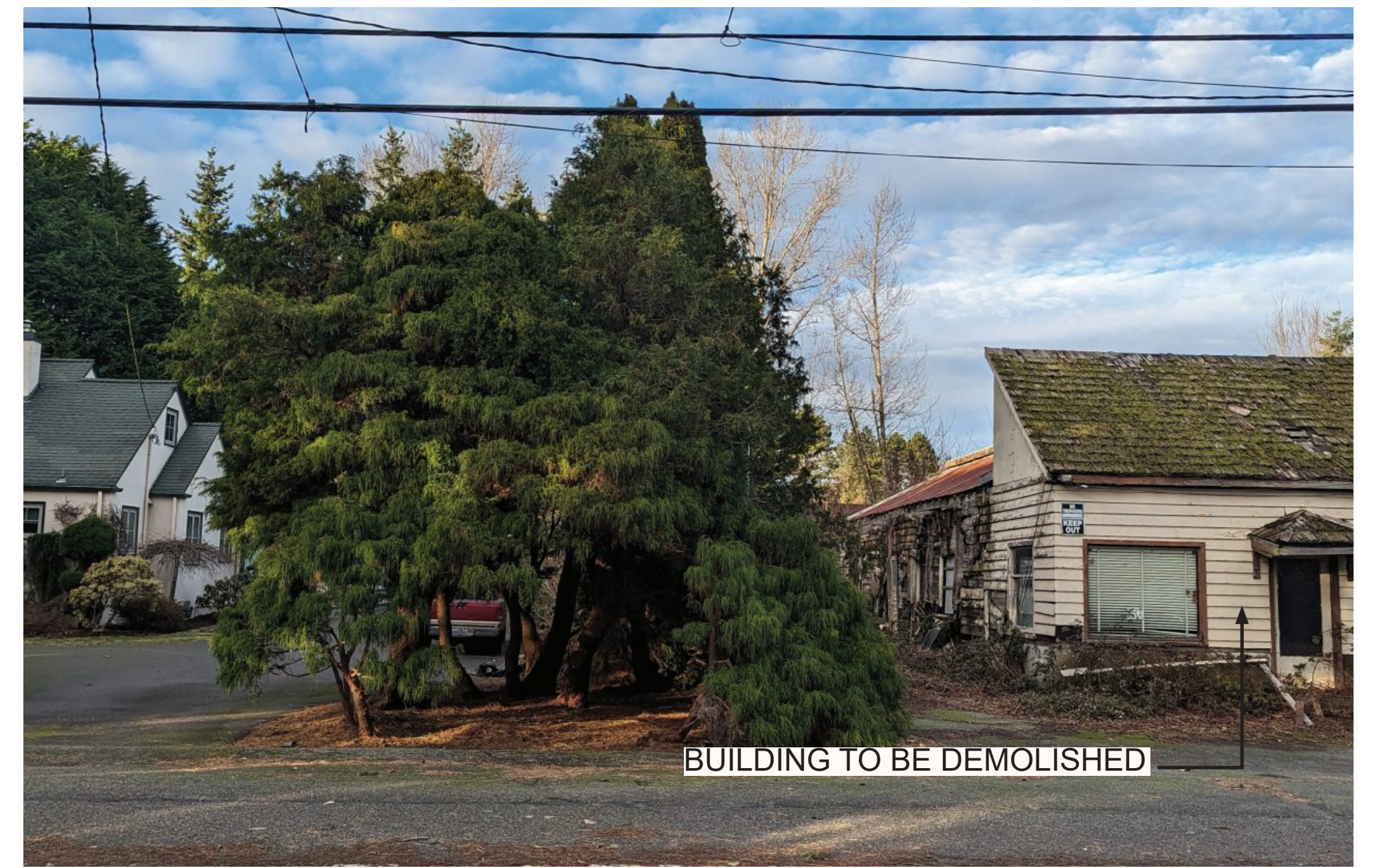
2. BIRCHWOOD STREET FRONTAGE
