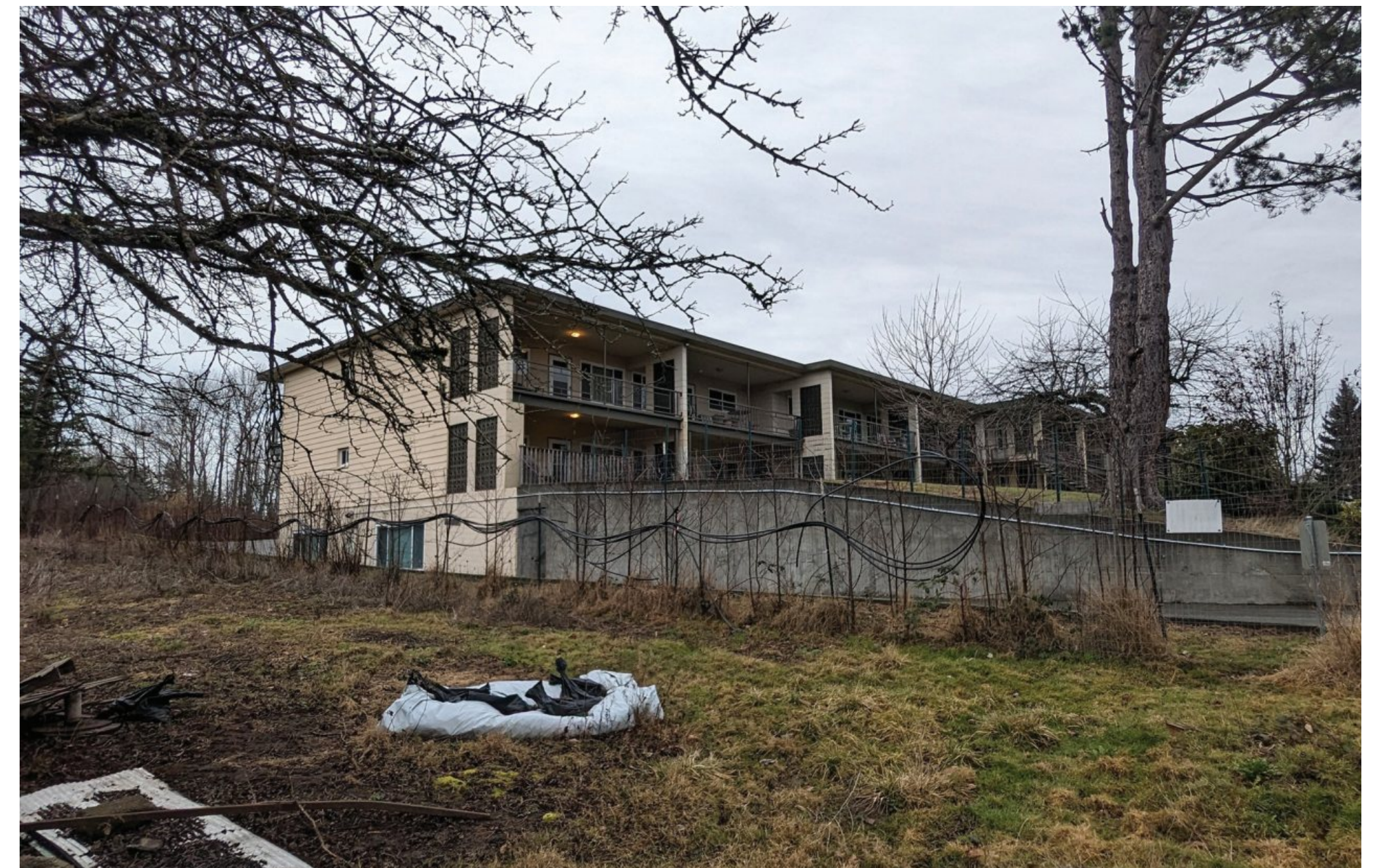
7. EXISTING APARTMENT COMPLEX
