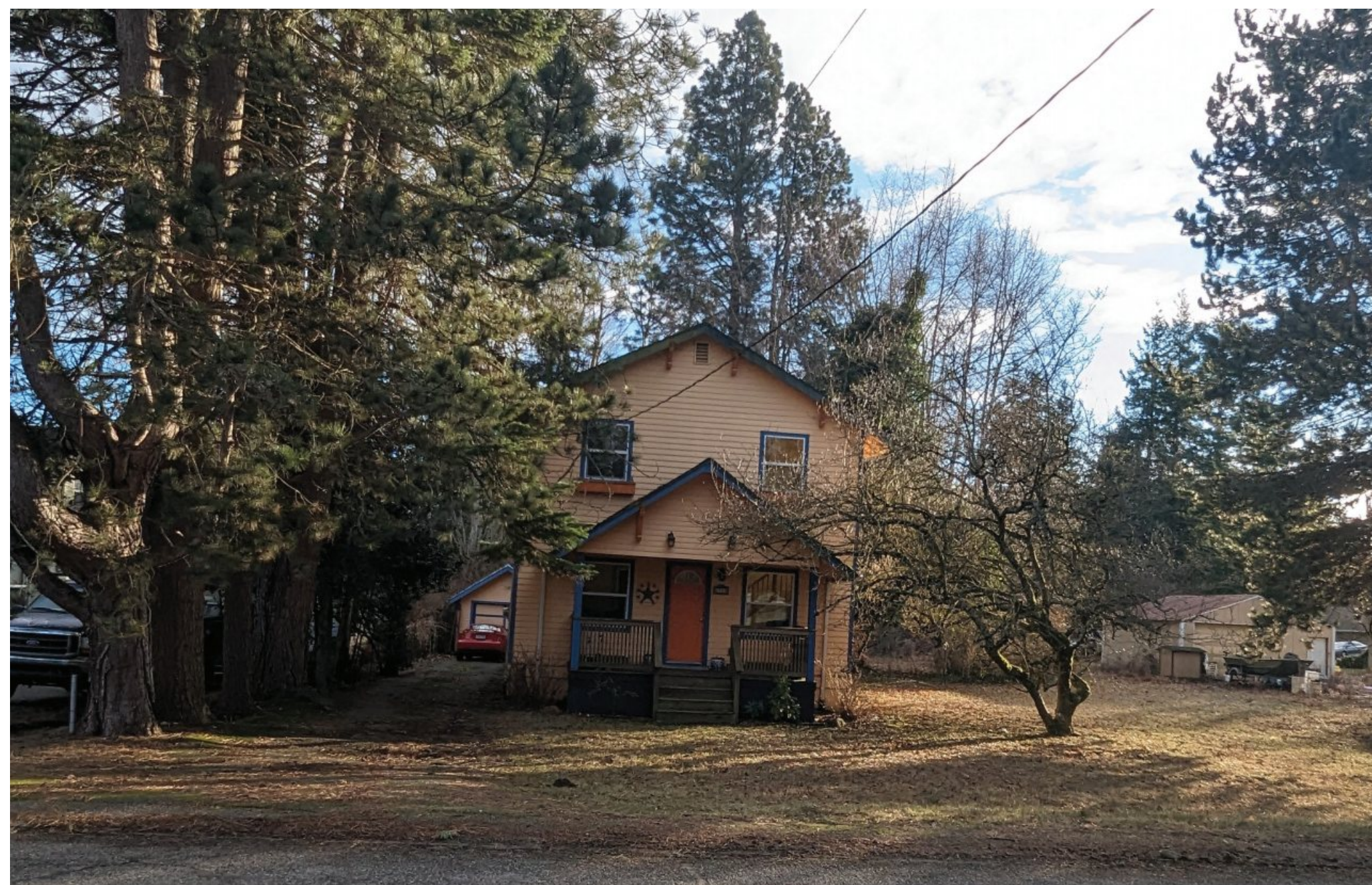
5. BIRCHWOOD STREET FRONTAGE
