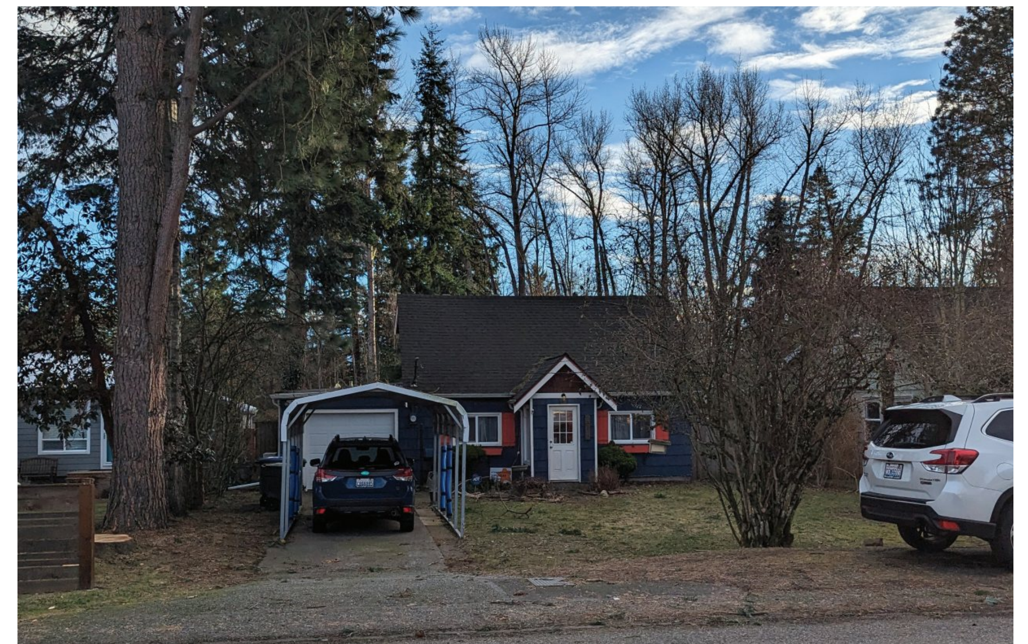
7. BIRCHWOOD STREET FRONTAGE
