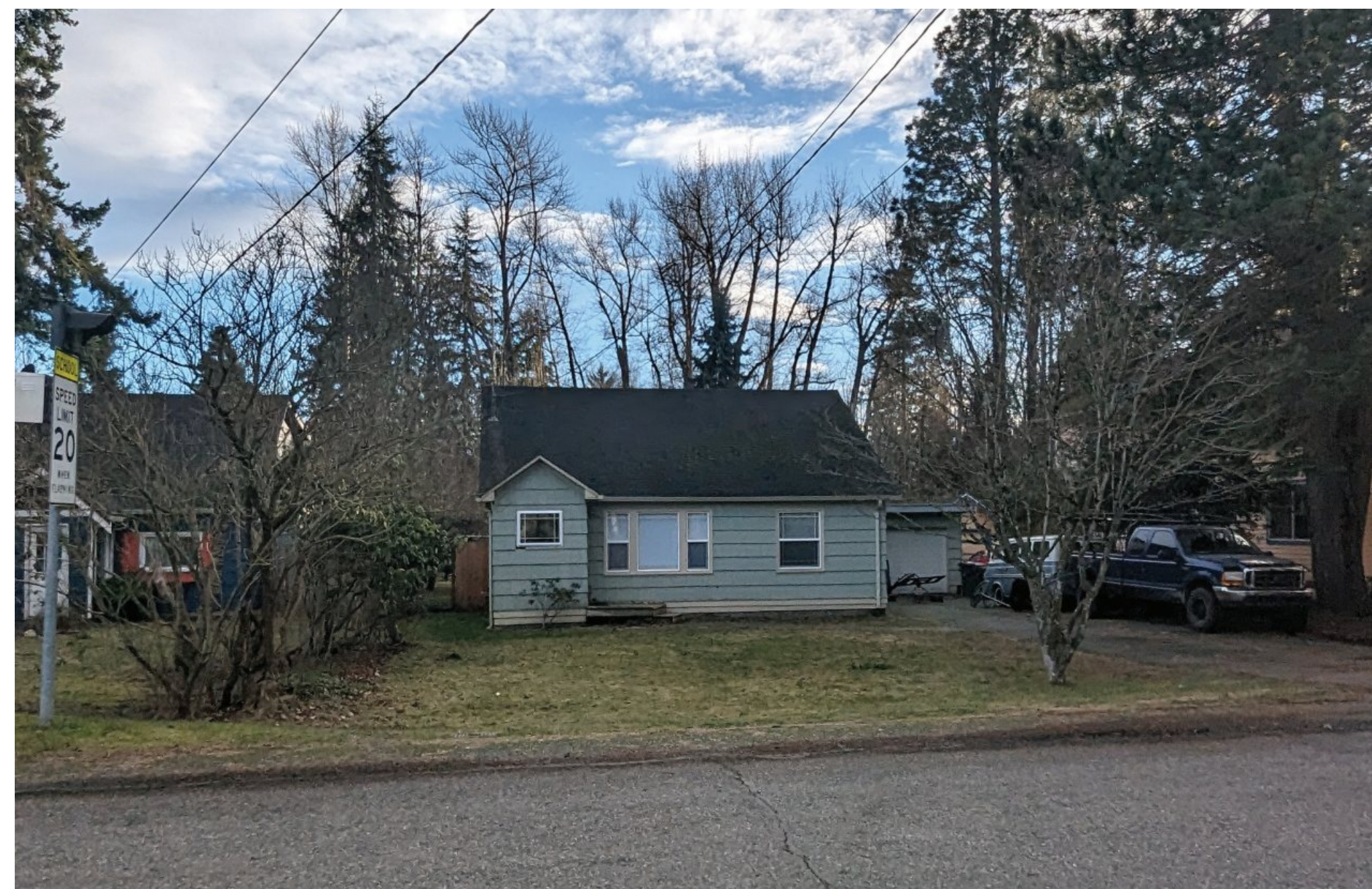
6. BIRCHWOOD STREET FRONTAGE
