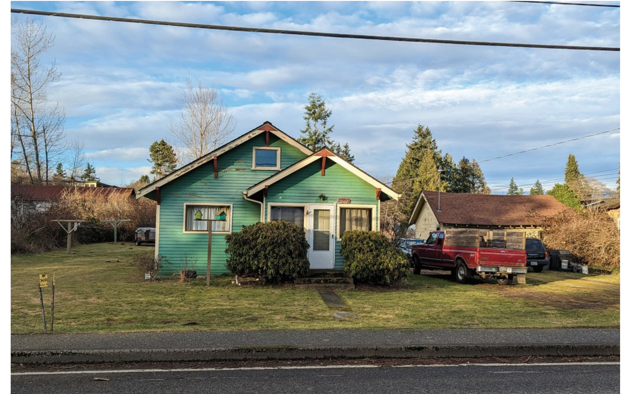
4. BIRCHWOOD STREET FRONTAGE
