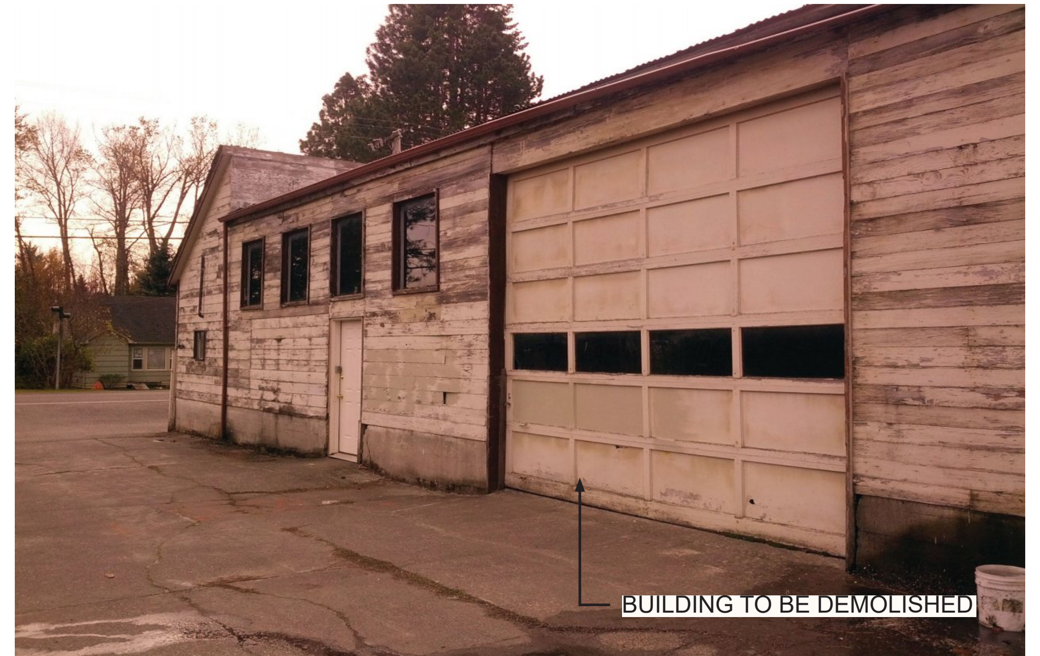
4. 2912 BIRCHWOOD - EXISTING ACCESS
